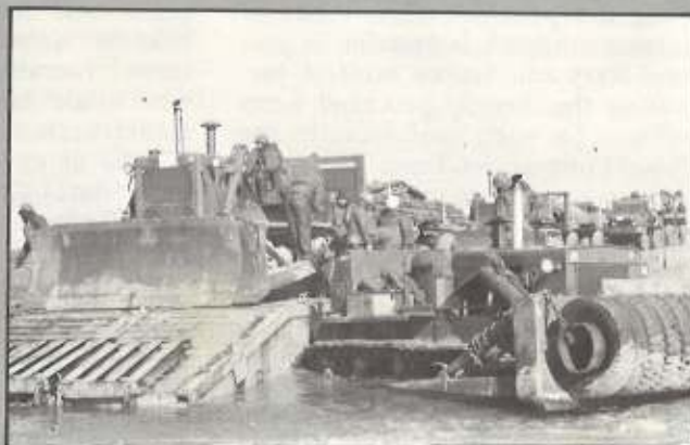
BARGE FERRY with bottom lay fuel system arrives at beach for Seabee installation.
