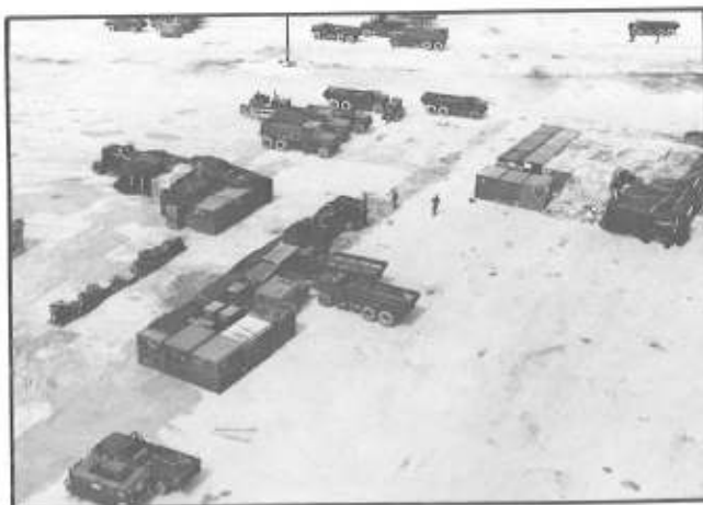
NMCB-40's equipment and rolling stock is positioned for simulated deployment to overseas site.
