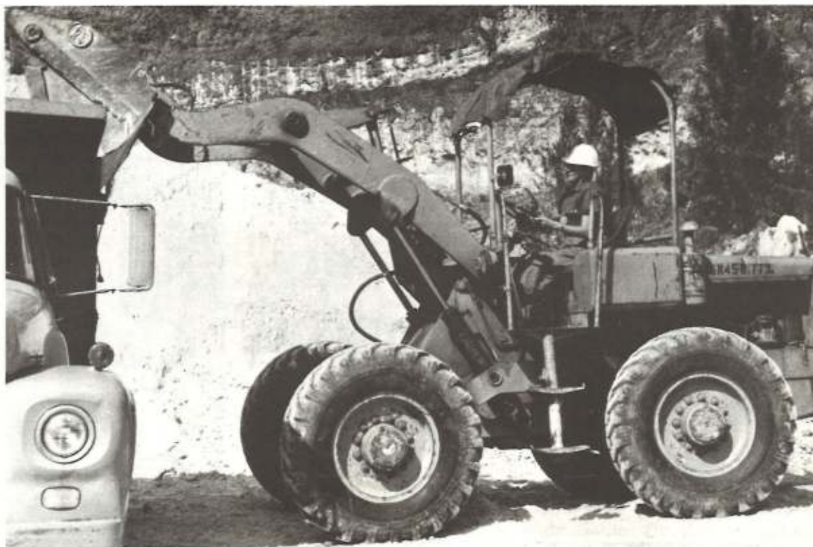
WOMAN POWER —Equipment Operator Second Class Viviana A. "Jo" Bailey, Naval Reserve Unit PWC Guam 119, takes to the gears of a front-end loader and drops a bucket
