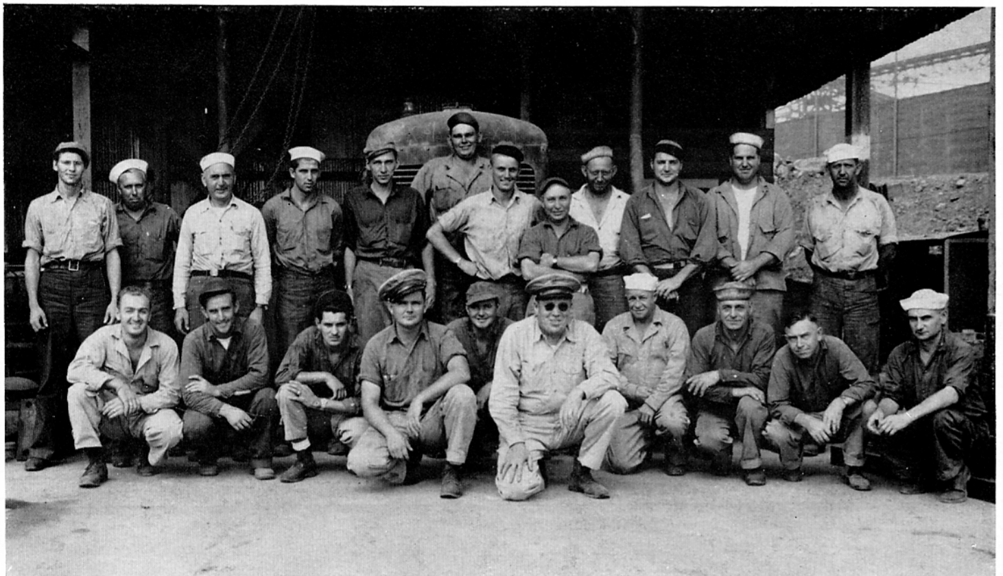
HEAVY EQUIPMENT REPAIR
