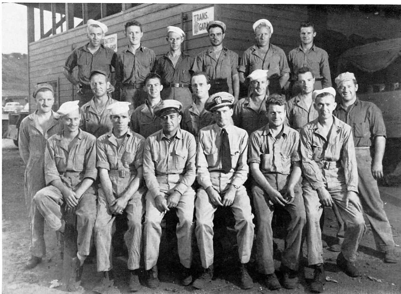
GARAGE REPAIR CREW
