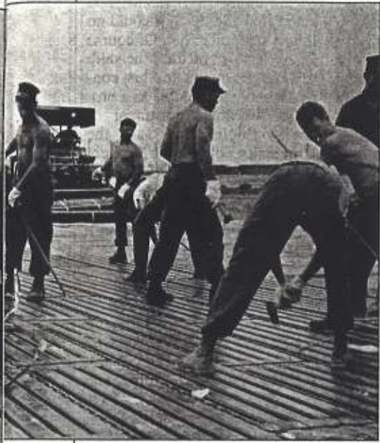
Seabees lay steel matting for airfield, Phu Bai, Vietnam, January 1968.
