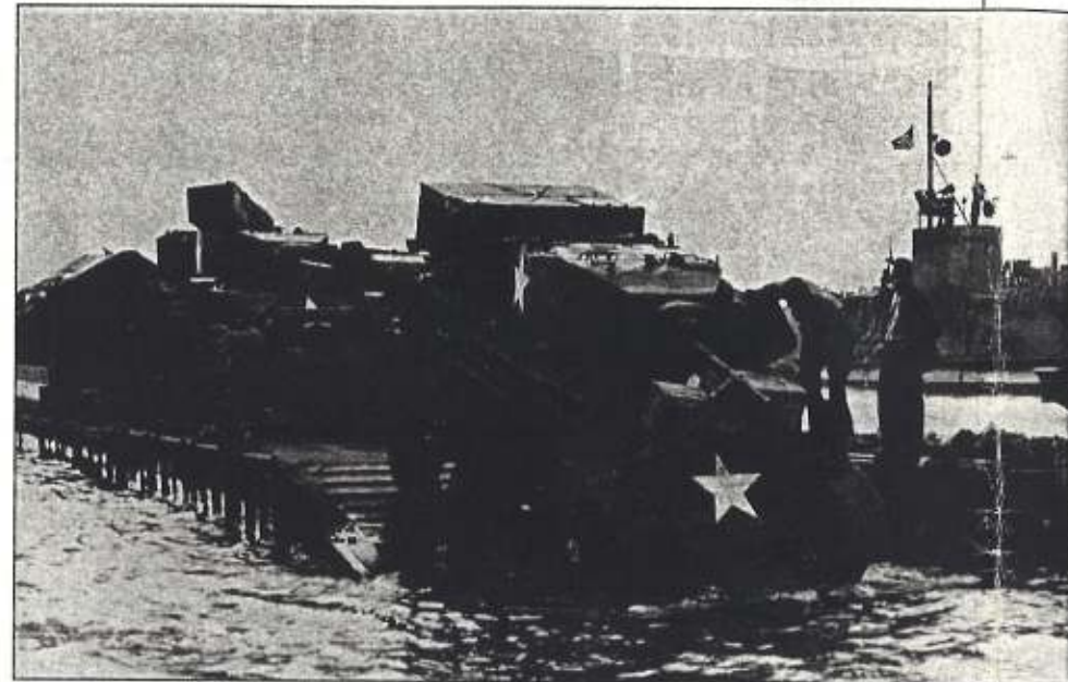
The 70th Naval Construction Battalion unloads tanks from a pontoon barge during the invasion of Okinawa, April 1945. The construction battalions, better known as "Seabees," comprise a famous and colorful component of naval history. Many AGC contractors and employees are Seabee veterans.
