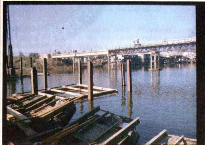
Dang Ha River Bridge Nov. 1969
